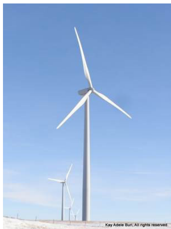
Source: Velva Wind Farm in McHenry County, ND. Courtesy of Kay Buri.
